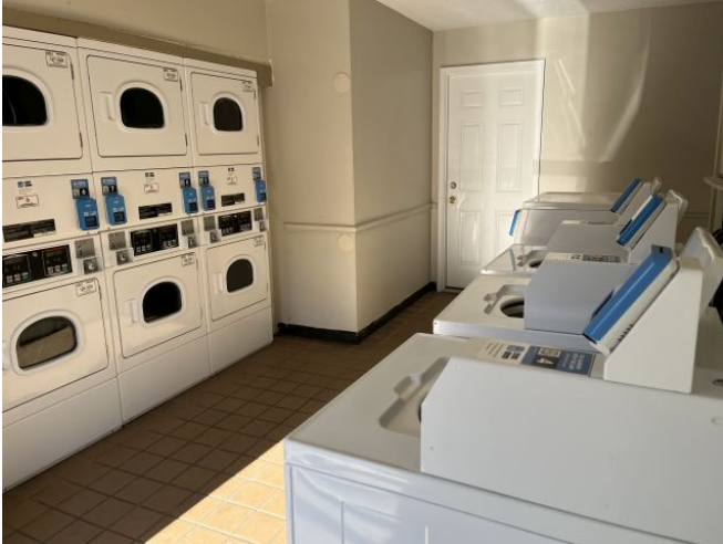
Subject's central laundry facility
